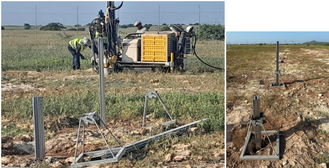
Photo 3 - Drilling for implementation of the panel structures on Maio Island (Source UGPE - MRV)
