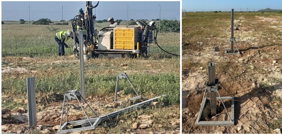
Photo 3 - Drilling for implementation of the panel structures on Maio Island (Source UGPE - MRV)
