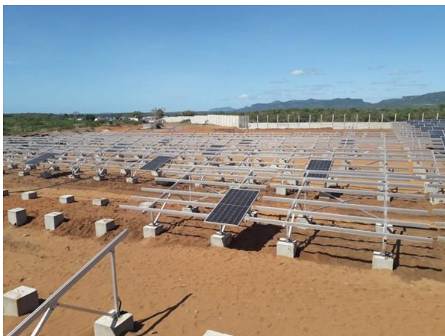
Photo 2 – Solar PV plant with aluminum structures and concrete blocks in Madagascar (Source MRV)
