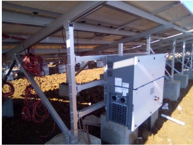
Photo 4 - Inverter installation on panel structures in Madagascar (Source MRV)
