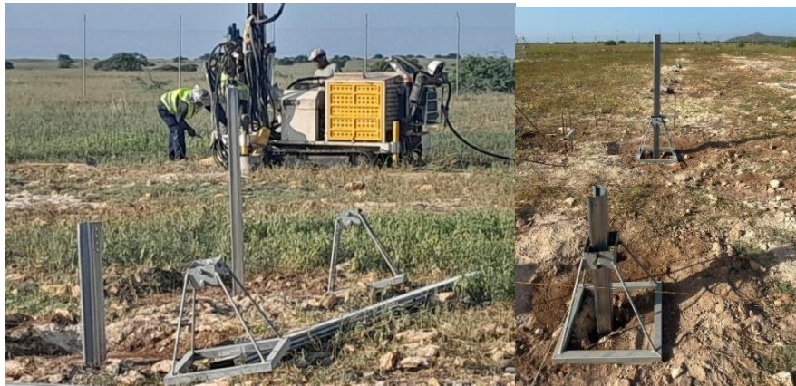
Photo 3 - Drilling for implementation of the panel structures on Maio Island (Source UGPE - MRV)
