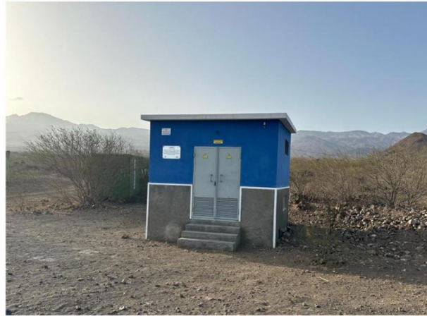
Photo 6 - Typical 20 kV Medium Voltage Substation in Cabo Verde (Source MRV)
