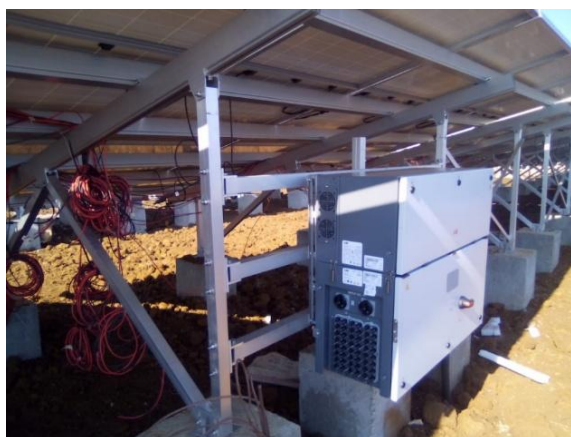
Photo 4 - Inverter installation on panel structures in Madagascar (Source MRV)
