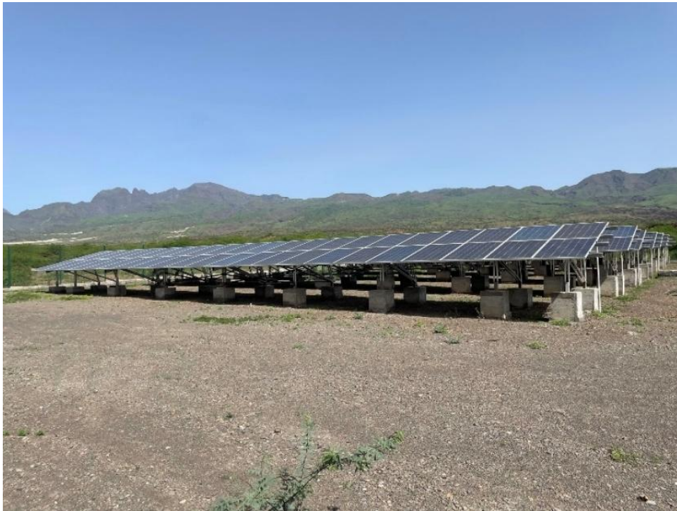
Photo 1 - Solar PV panels and support structure set in concrete blocks (Santo Antão Island) (Source MRV)
