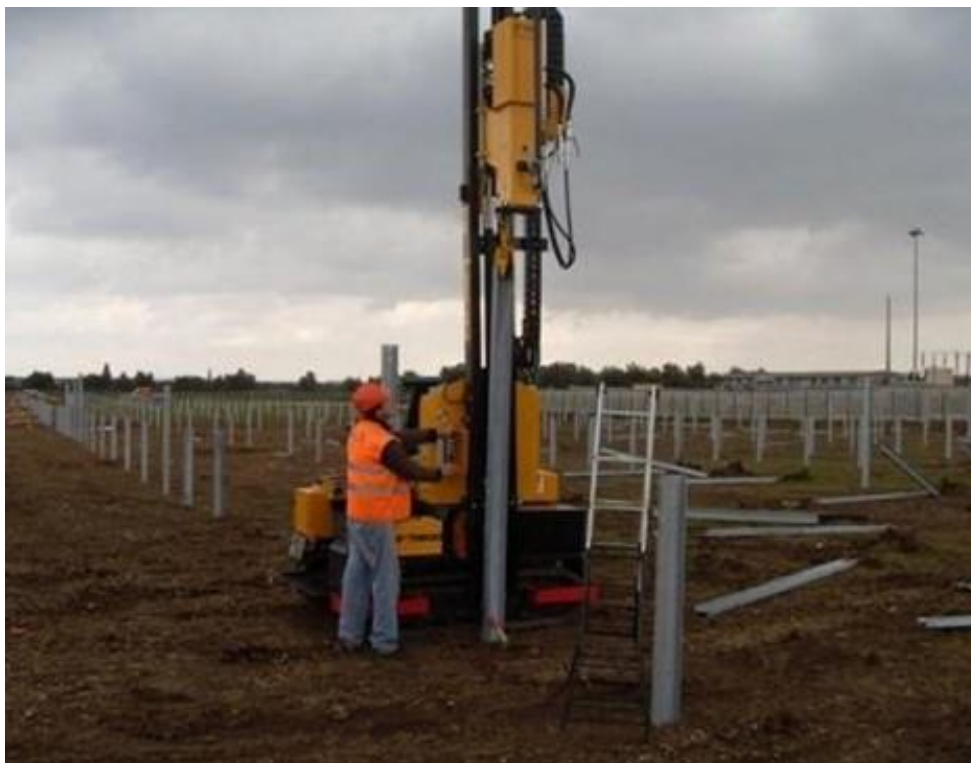
Photo 4 - Driving of metal profiles for the foundation of the structures
