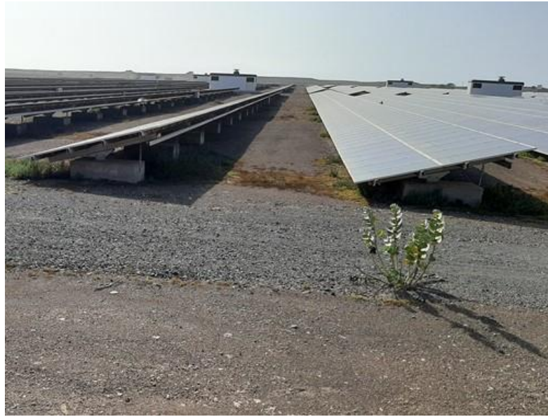
Photo 2 - Solar PV panels and support structure set in concrete blocks (Sal Island)
